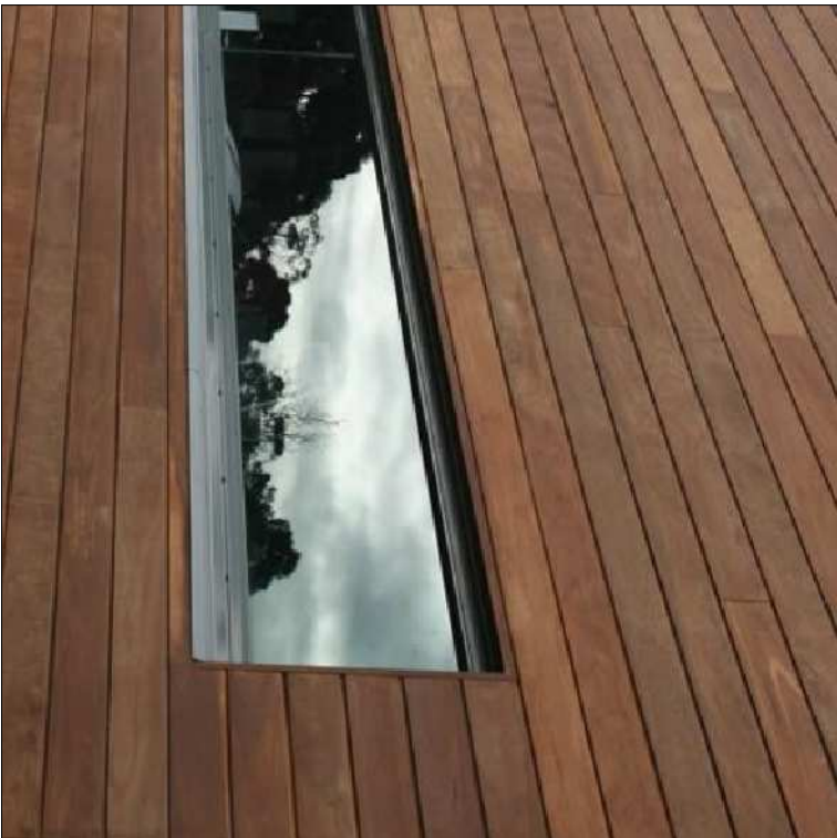
HORIZONTAL TIMBER CLADDING
