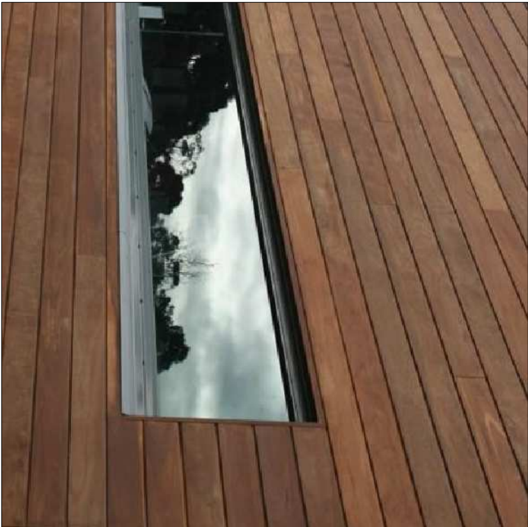
HORIZONTAL TIMBER CLADDING
